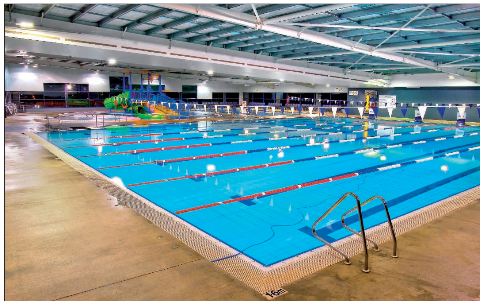
ABOVE: Geelong Bellarine Aquatic Centre to include indirect evaporative cooling.
