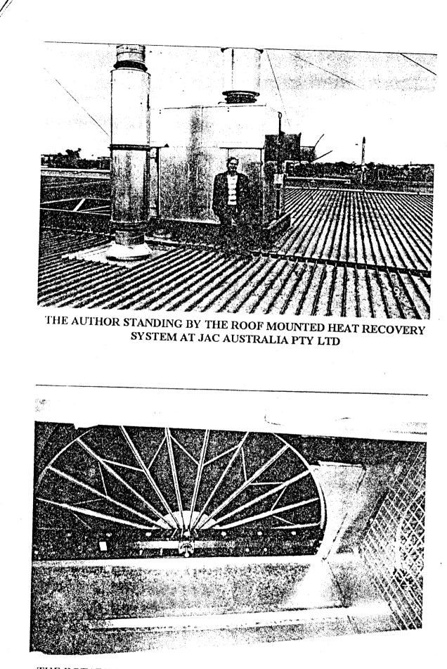
THE ROTARY HEAT WHEEL INSIDE THE PLENUM CHAMBER WHICH SEPARATES THE EXHAUST FROM THE HEATED FRESH AIR
