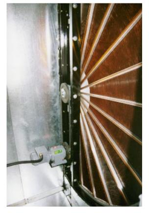
The interior of the rotary heat exchanger as used in the adhesive labelling dryer at Jac Pty Ltd.
